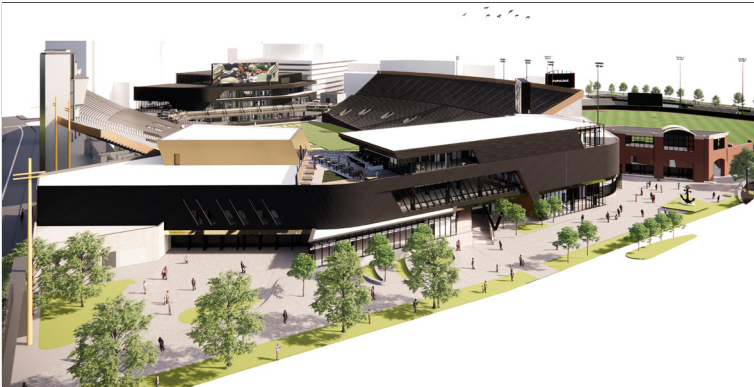
Exterior rendering of the competed renovations at FirstBank Stadium.
